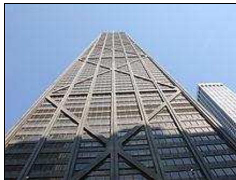
Fig 2 Cross bracing
